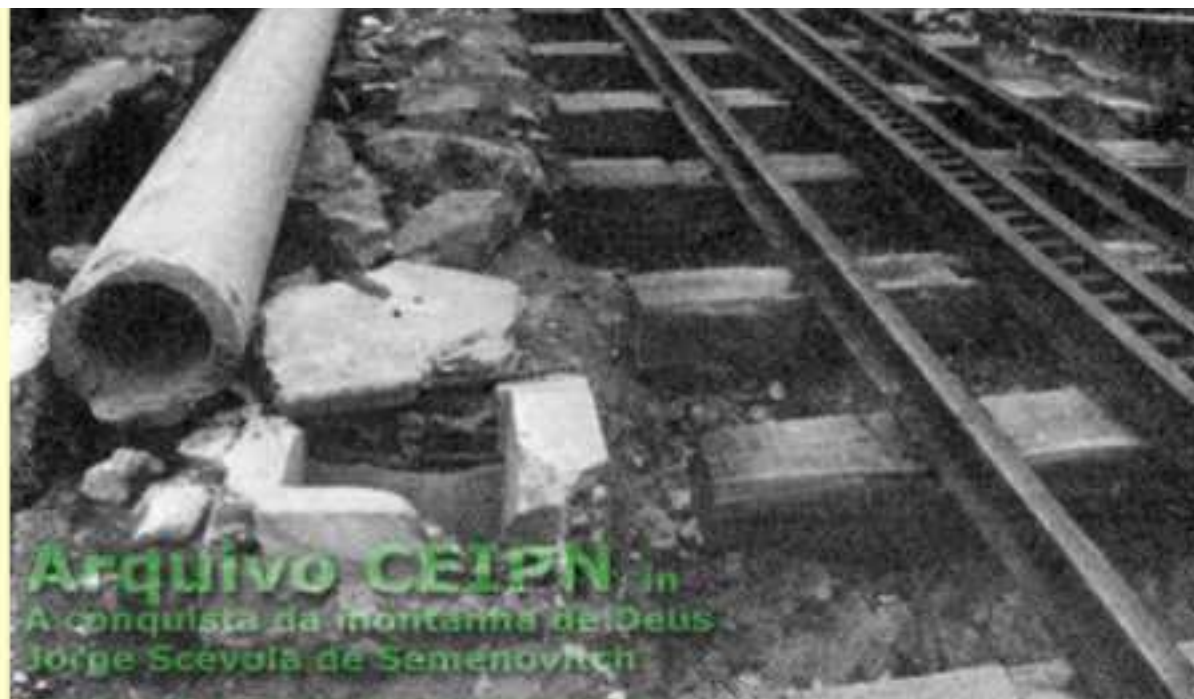
Settlement of new rails, racks, sleepers and poles of the Corcovado railway, in Silvestre
