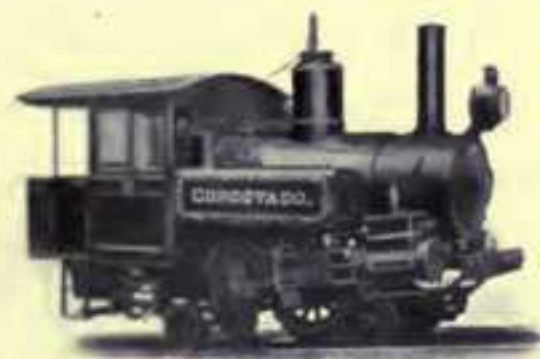
RACK LOCOMOTIVE, RIGGENBACH SYSTEM
